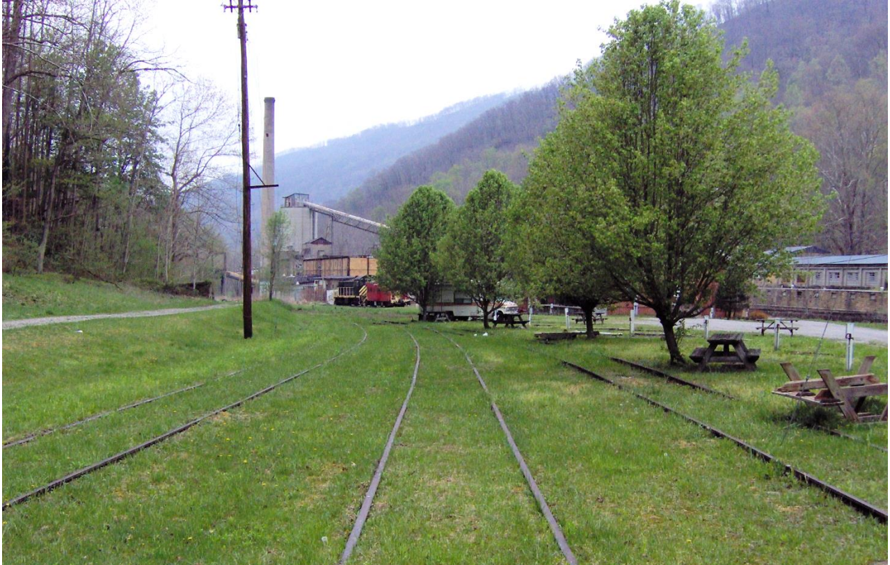
Looking South toward Benham with the Existing Campground to the right and the “Largest Coal Tipple in the United States” when constructed and is visible in the foreground of this photo.
