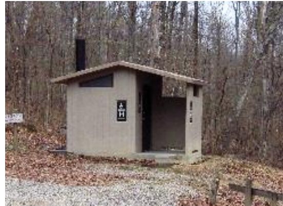
Vaulted Toilet beside proposed “Field” Campground
